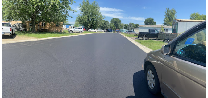
Beautiful new road surface at Sungold Heights Cooperative- ready for roller skating!
